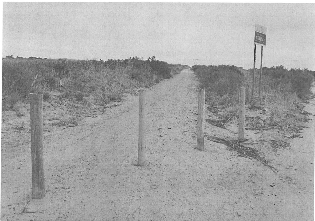
Jeep track which was successfully cordoned off by the municipality in the past using gum poles as bollards
