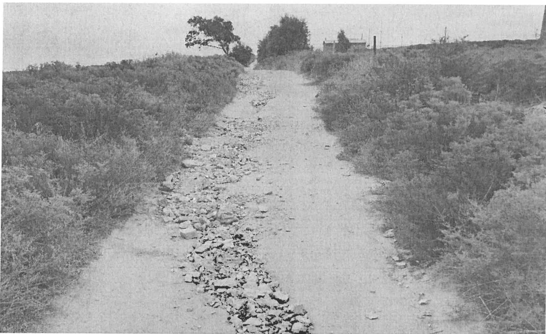
View of Jeep Track leading to Eskom Distribution's Klipfontein Substation showing infilling with building rubble
