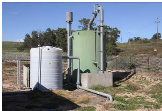
Rapid gravity sand filter for supply from Paardenberg Dam
