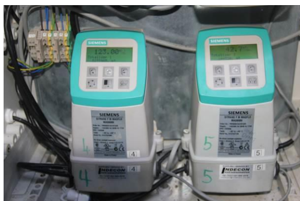
Siemens bulk water meters at Kleindam reservoirs
