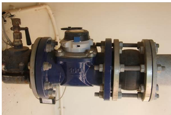
Riverlands/Chatsworth Supply PS bulk water meter, 100mm dia., (Sensus) at Kalbaskraal
