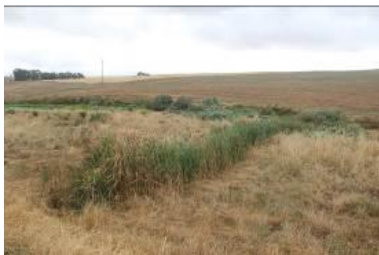
Overflow from last secondary pond
