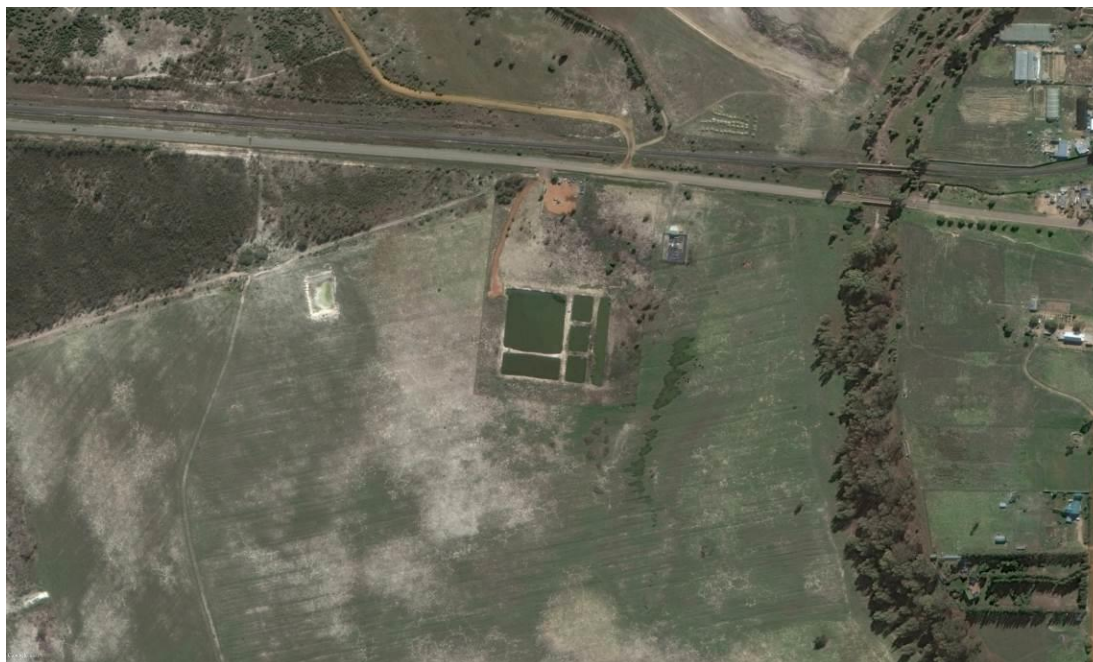
Figure 2: Aerial photo of the Kalbaskraal WWTW
