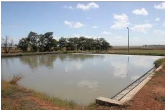
Anaerobic Pond No.1
