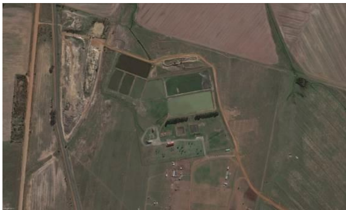
Figure 2: Aerial photo of the Darling WWTW
