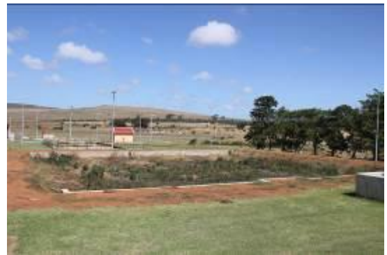
Anaerobic Pond No.2
