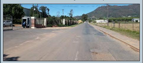
**Lelie Street:** is a classified Class 4 collector road (width ±6.6m). It is a two-lane undivided road (one lane per direction) with no shoulders. There is no posted speed limit along Lelie Street in the vicinity of the site. A paved sidewalk is present along the eastern side of the road.
